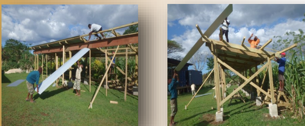
Figure 8: Construction timber drying shed at TRF
